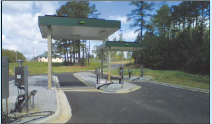
Figures 6 & 7: The Completed Unloading Area
