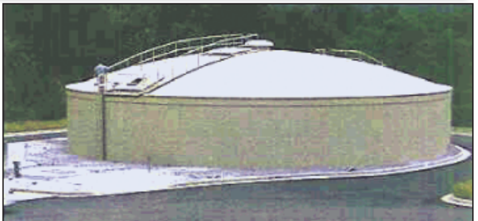
Figure 8: Completed Grease & Septage Storage Tank
